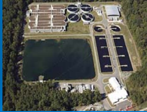
Durham County North Carolina WWTP
